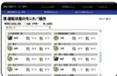
Control computer for the centralized air conditioning management system
